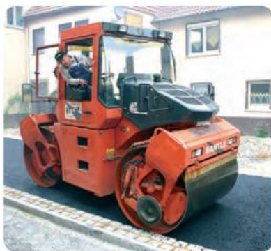
A steamroller being used in street construction.
